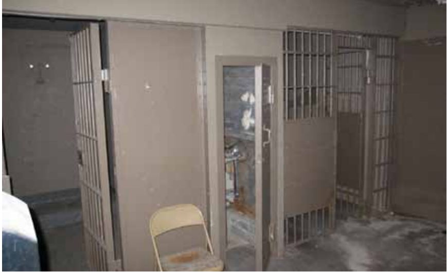
Central area of basement jail
