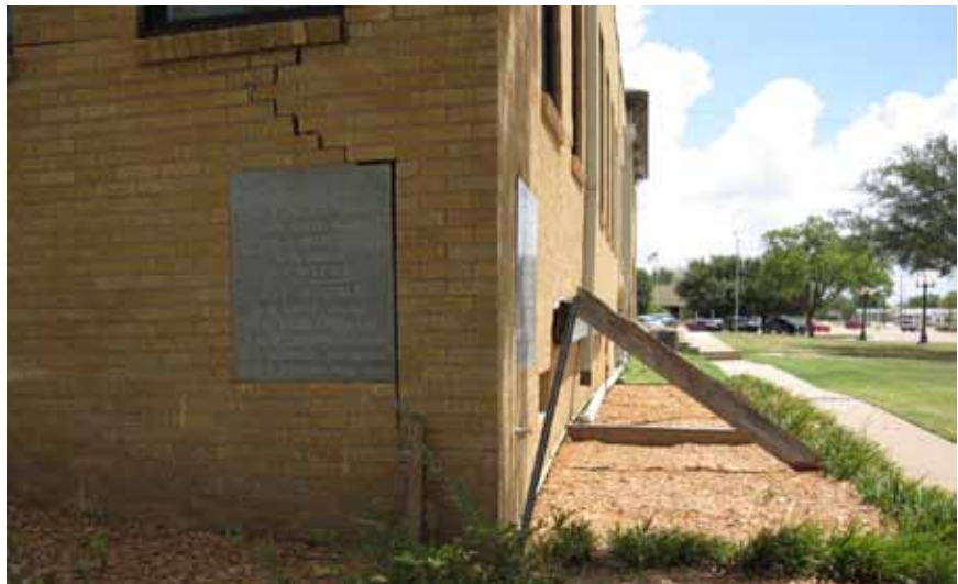
Wood supports on the south wall
