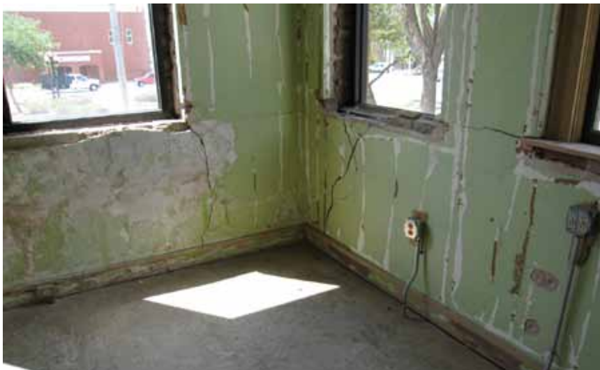
Windows and floor at former Police area
