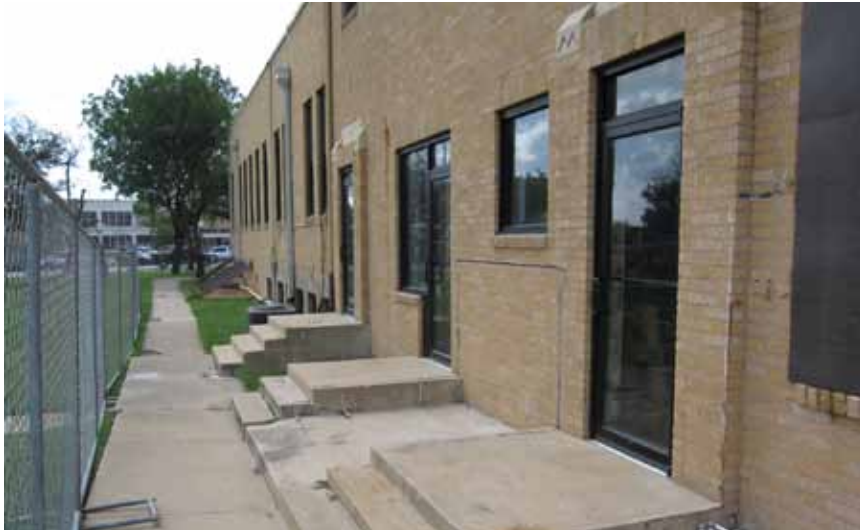
South wall of former Fire Station
