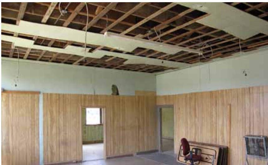
Main office of former Police area
