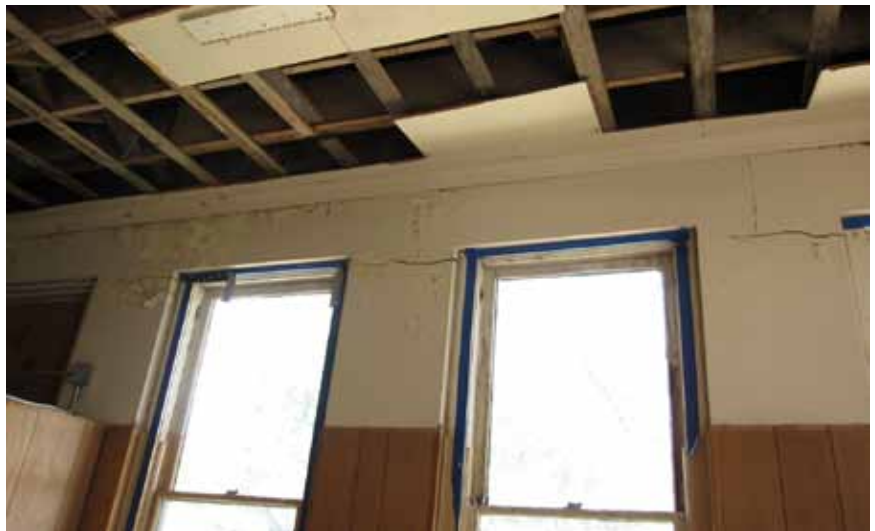
Wall, window and ceiling in former Police area
