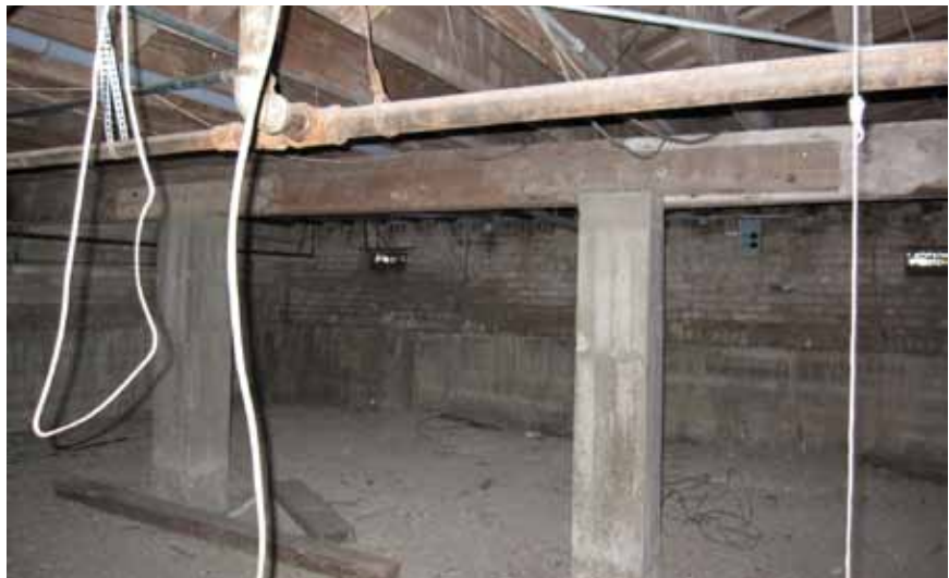
South portion of crawl space showing concrete supports
