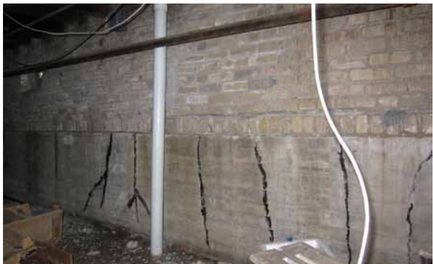
Crawl space showing south wall cracks
